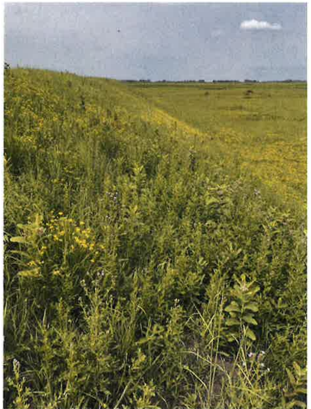
North embankment outside slope
