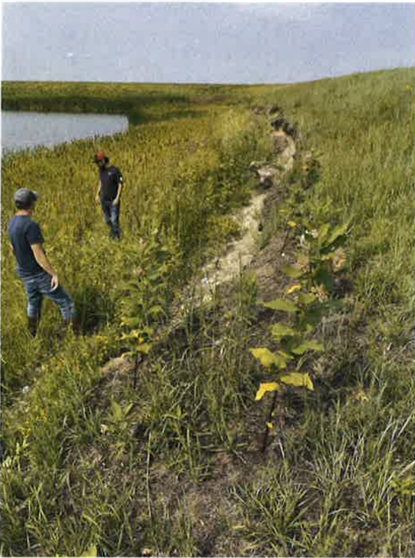
North embankment inside slope
