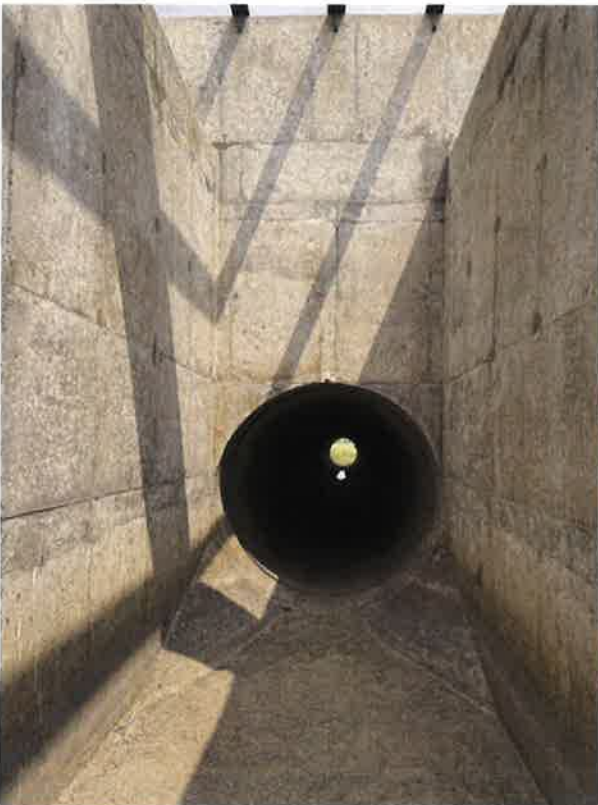
Principal spillway riser
